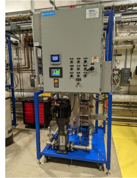
Above right: New L4 water skid
