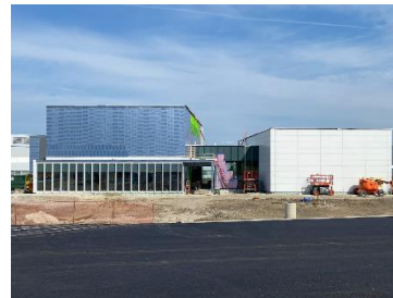
Long Beamline Building progress
