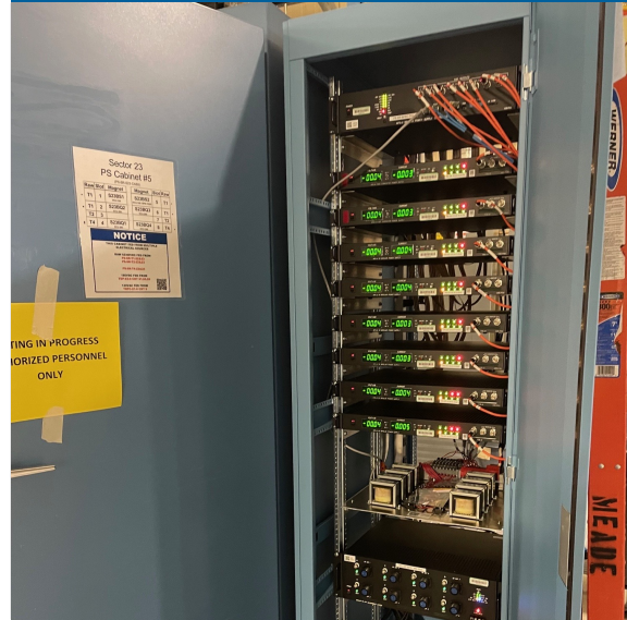
Test and checkout
